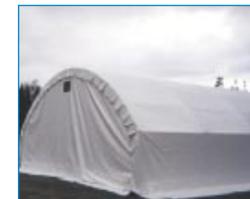
Structure tunnel 8 x 12 m.
